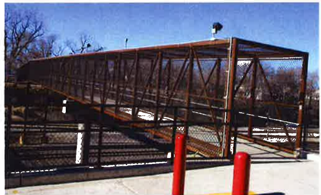
Restored Pedestrian Bike Bridge
