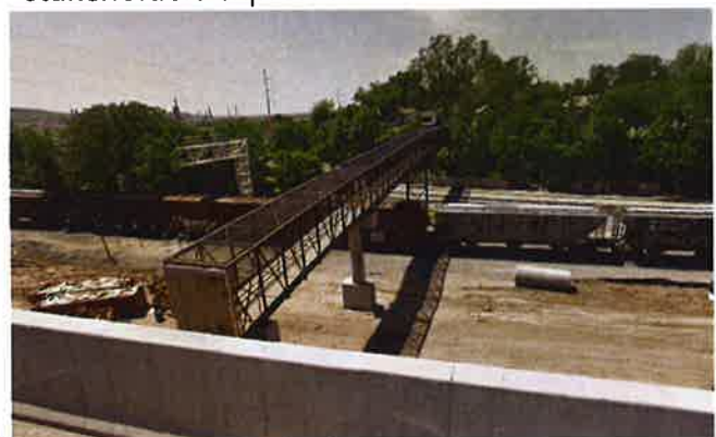
Pedestrian Bike Bridge, closed for reconstruction.
